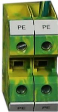
Figure 6: Ground Bus Terminal Blocks
