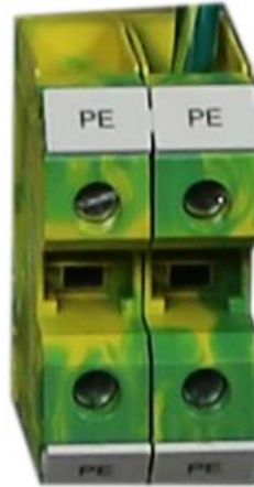
Figure 6: Ground Bus Terminal Blocks
