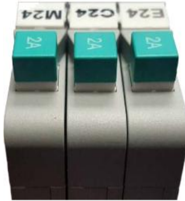
Figure 75: Breakers in the OFF Position
