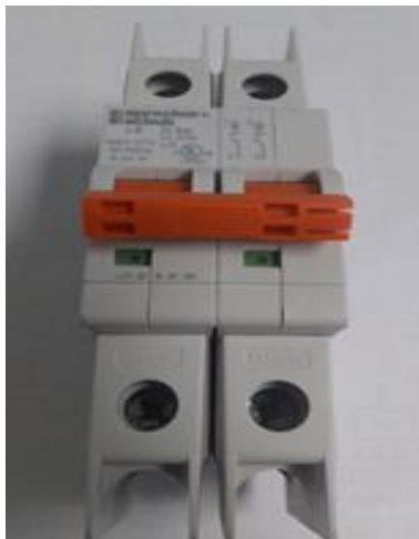
Figure 116: L1/L2 Breaker
