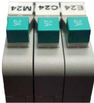
Figure 115: Breakers in the OFF Position
