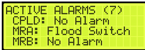
Figure 717: Active Alarms Menu
