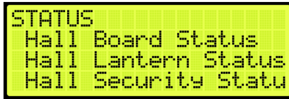
Figure 49: STATUS Menu – Hall Security Status
