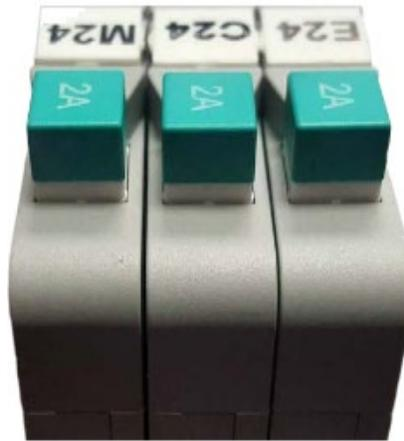
*Figure 35: Breakers in the OFF Position*
