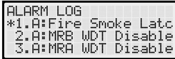
Figure 207: ALARM LOG Menu
