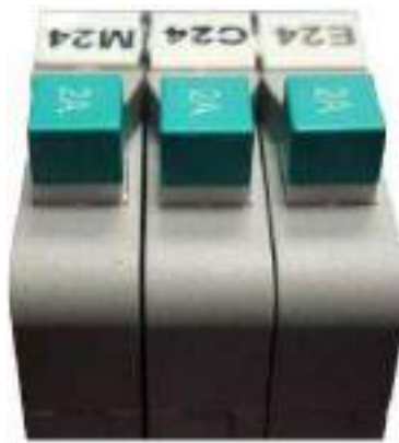
Figure 115: Breakers in the OFF Position
