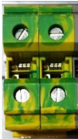
Figure 3: Ground Bus Terminal
